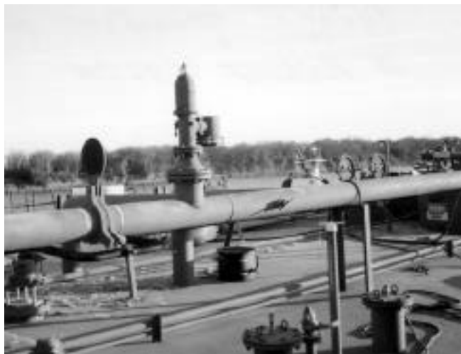
Typical PV Valve Installation
